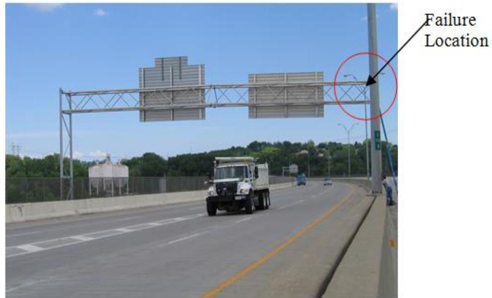
The location of a failure was adjacent to the end of the girder truss, at the weld between the branch and chord member after 36 years.
