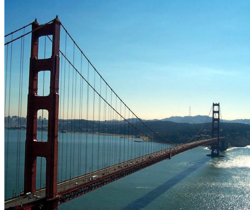
Golden Gate Bridge (San Francisco)
